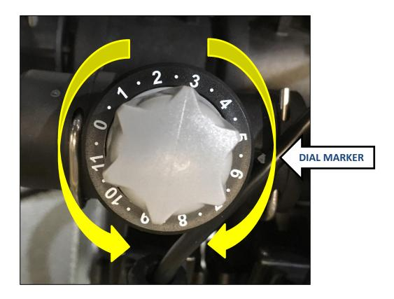
5. Repeat step 4 for remaining valves one at a time. Sections with the same number of outlets will normally end up with the same setting on the dial.
